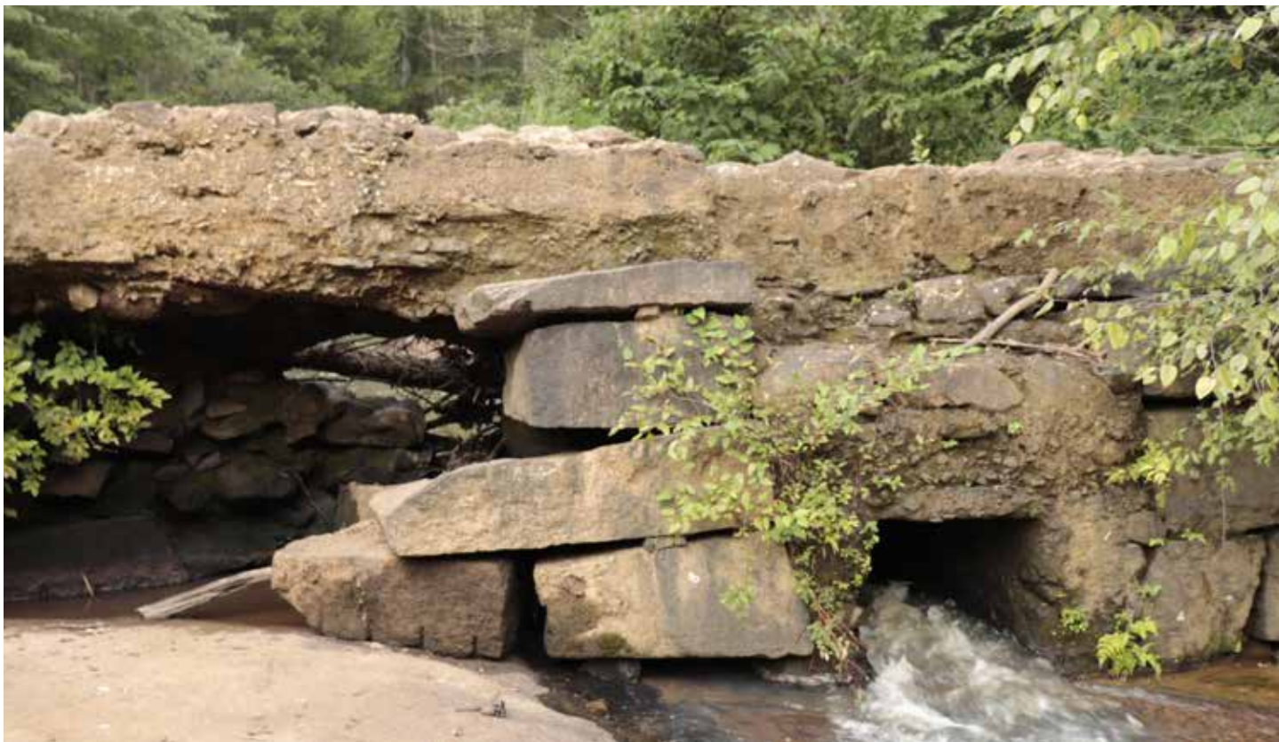
The dam at the Berry Cochran Mill site has been compromised in several places. Vegetation is allowed to overgrow the structure.
