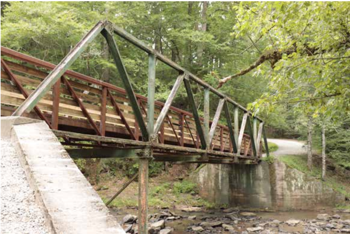
The remains of the historic bridge with the new pedestrian bridge fitted into place.
