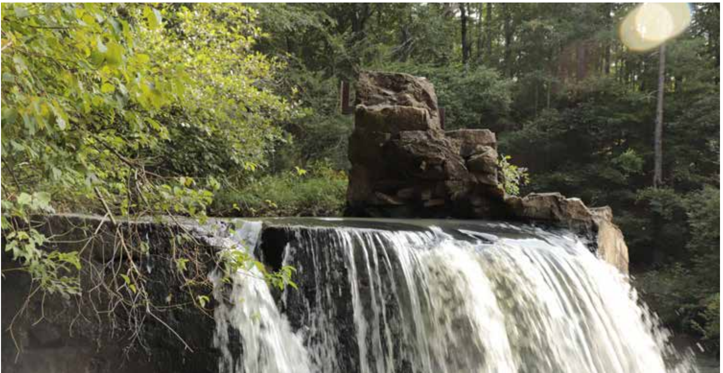
The concrete dam constructed by Blalock has been breached in order to drain the lake.
